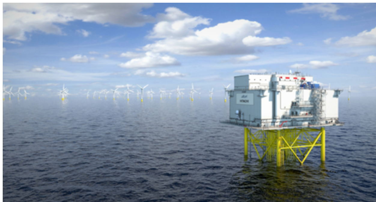
FIGURE 5. An offshore converter station at Dogger Bank, United Kingdom
