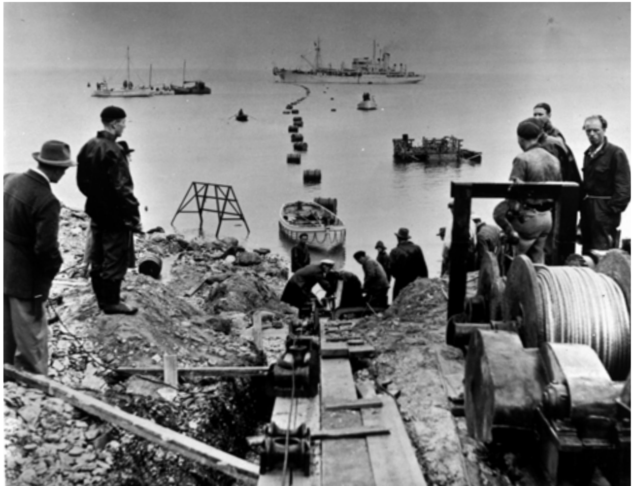
FIGURE 4. Gotland HVDC Link
