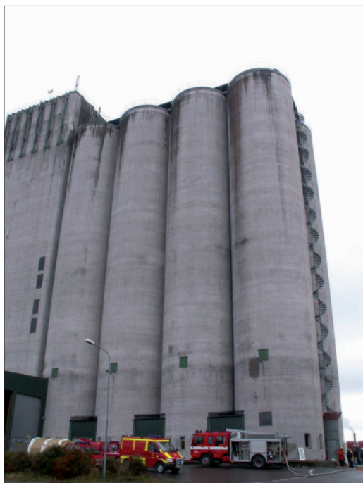
Figure 3.18. Mobile fire fighting unit for silo fire fighting. Example of 47 m high silo (left) fire successfully extinguished in Sweden 2007 by injection of nitrogen using mobile equipment (right) consisting of a vaporisation unit and a tank for liquefied nitrogen; [141].
