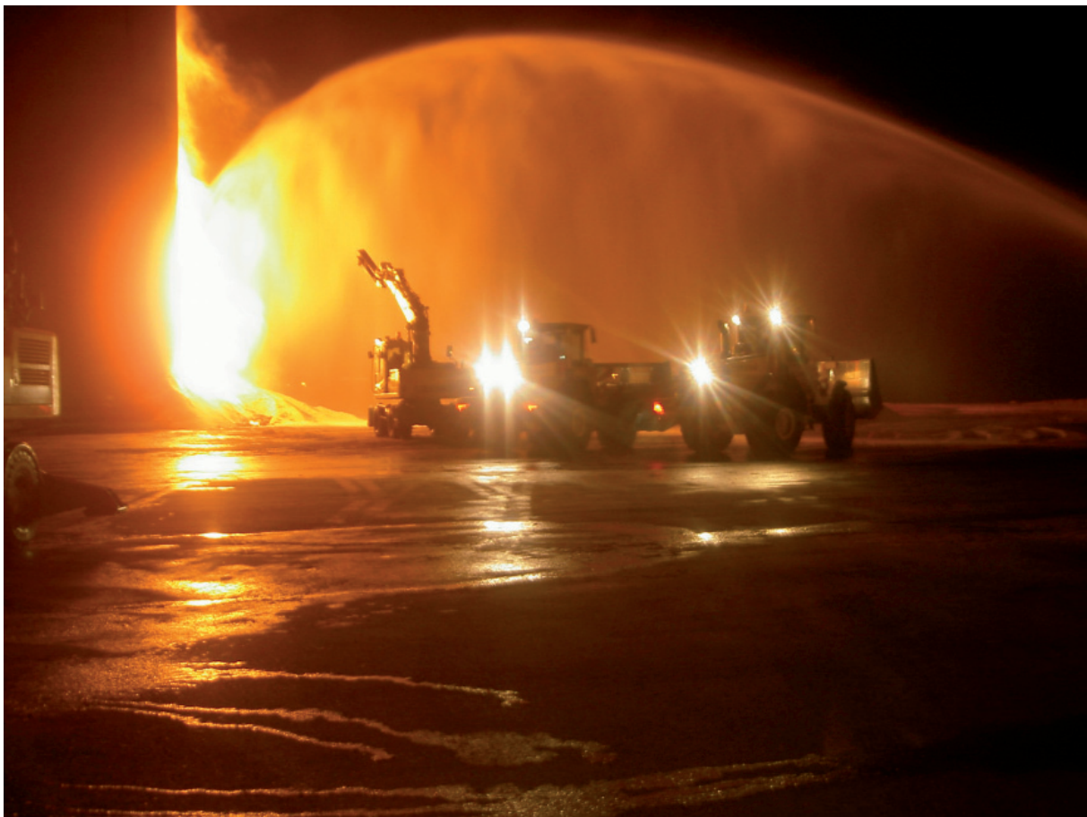
Figure 3.21. Flames on the outside of a silo caused by an opening in the silo wall [8].
