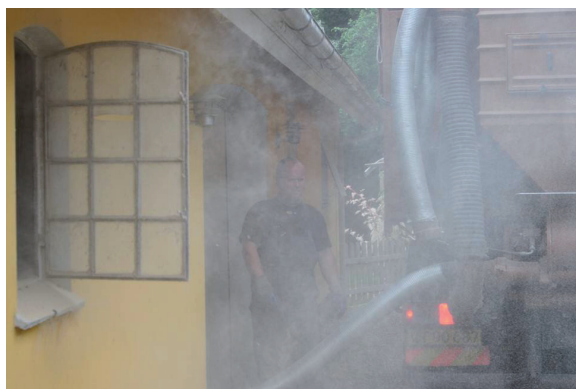
Figure 8.6. Heavy dust load around the truck by wood pellet delivery to private household, see Figure 8.5. The silo in the house is without cyclone which means that the transport air has to escape through the open window in the yellow wall. This causes the heavy dust load around the truck and the driver [158]
