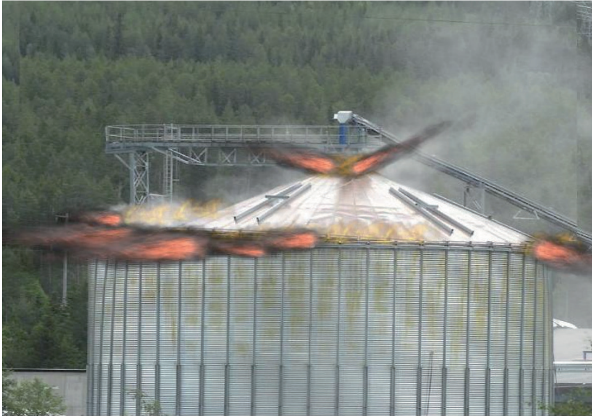
Figure 3.2. A real silo explosion which most likely occurred due ignition of headspace gases by an electrostatic discharge in an attempt to extinguish a smouldering fire. (courtesy of Dag Botnen, Hallingdal brann- og redningstenste iks, Norway)
