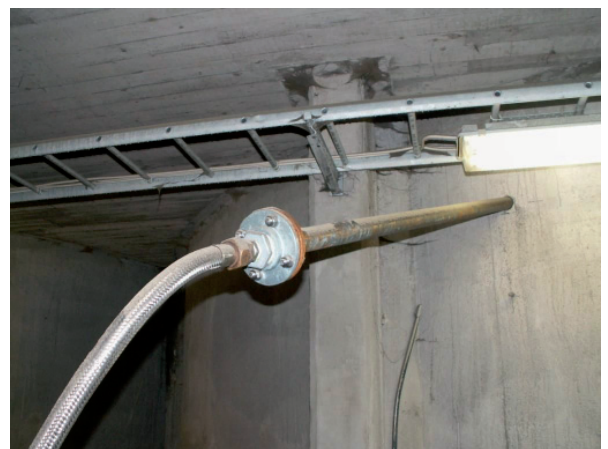
Figure 3.20. A 50 mm perforated steel pipe (left) used for gas injection in a silo fire in Sweden 2007. The lance was inserted through a drilled hole (right) close to the silo bottom and connected to the vapourisation unit by a hose; data source [141].
