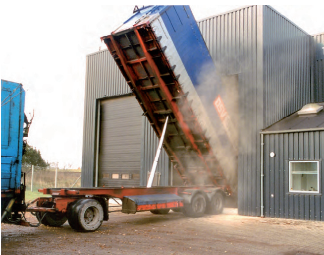
Figure 8.1. Wood chips unloaded at a Danish district heating plant. Very high concentrations of mould spores may prevail around the truck and inside the store during unloading, requiring personal protection for employers [157].
