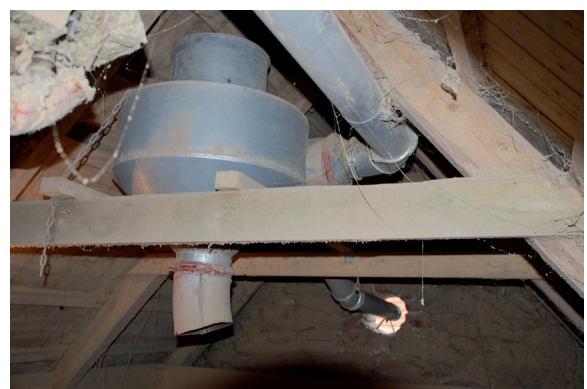
Figure 8.7. A better way to deliver pellets to a private end user compared to Figure 8.6. The pellets are blown from the truck in the pipe at the top of the picture and delivered to the silo through the open pipe in the bottom of the cyclone. The transport air is separated from the pellets in the cyclone and is blown in a tube through the hole in the wall to the open air far away from the truck and the driver [158].
