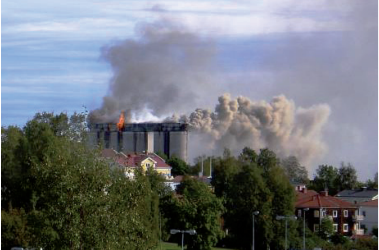
Figure 3.9. Fire in silo storage of wood pellets. (Courtesy of the Fire and Rescue Service in Härnösand, Sweden)
