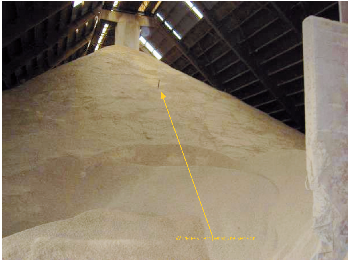
Figure 3.14. A pile of pellets in a flat storage. A wireless temperature monitoring spear is used for temperature control. To the bottom right, a separating concrete wall is also visible, which acts as a fire barrier in case of a fire incident.
